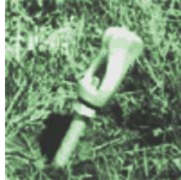
Unmarked Ground Anchor hiding Creep
